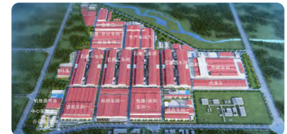
Construction of the integrated base for lithium-ion battery anode materials of Shanghai Shanshan Lithium Battery's Sichuan Plant
